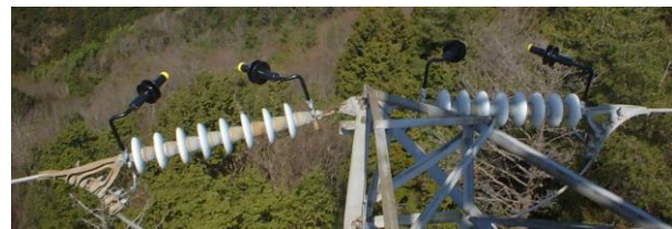
Fig. 1: Appearance of existing FCIAH
